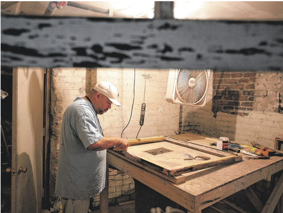
Charles Luna uses Bondo to restore window frames in the Wellsport Portwell Flats, two historic buildings in Des Moines’ Sherman Hill neighborhood. Most of the 120 windows in the buildings were rebuilt rather than replaced. Developer Jack Hatch is renovating the “twin sisters.” MARY CHIND/THE REGISTER
